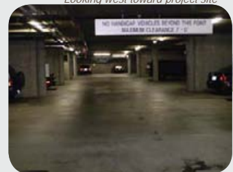
Internal garage conditions
