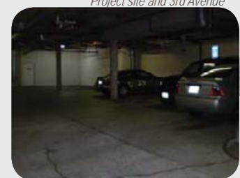
Internal garage conditions
