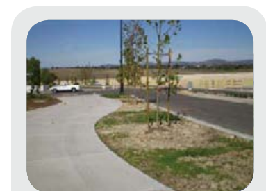
Northeast corner of project site
