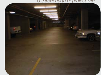
Internal garage conditions
