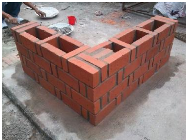
Figure1. Rat trap bond mechanism
