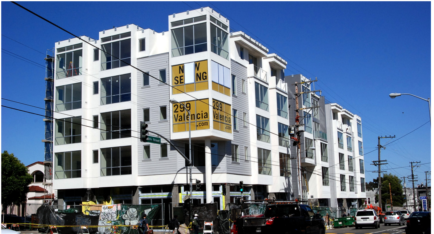
New construction at 299 Valencia added 36 units to the Mission District
