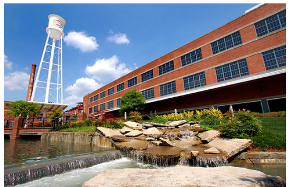
The American Tobacco Campus in Durham, NC was revitalized with the help of New Market Tax Credits. 16
