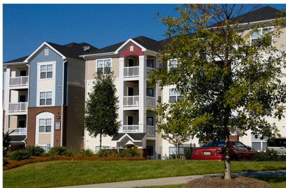
South Oak Crossing Apartments in Charlotte, NC. 39
