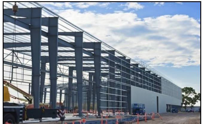
Fig -4: Industrial Construction
