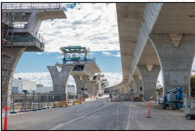
Fig -3: Infrastructure Construction
