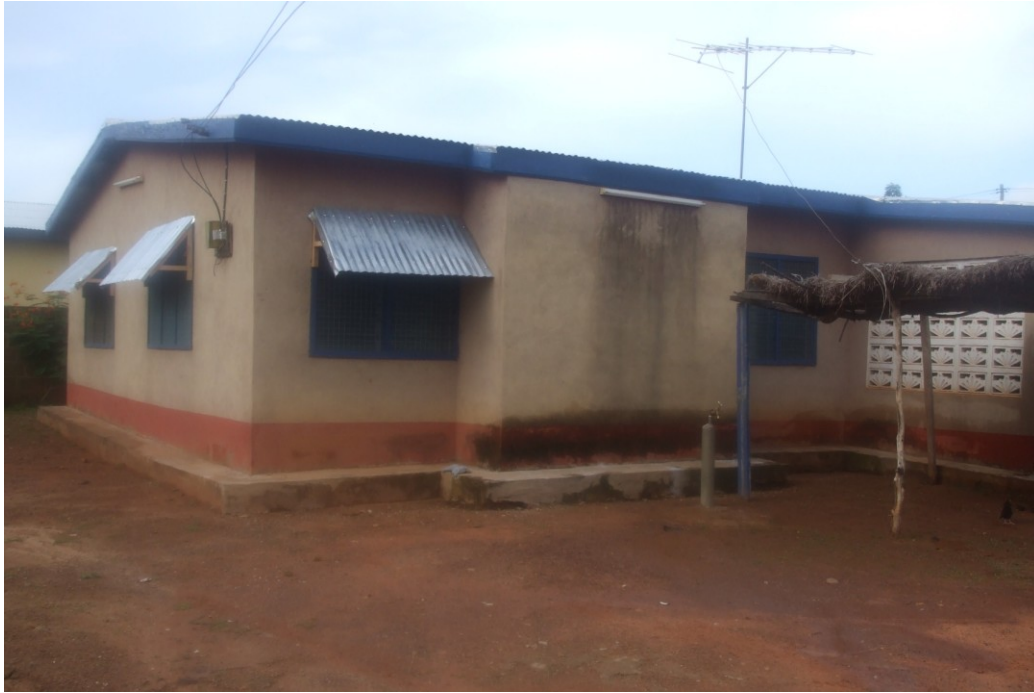
Plate 4.8: High quality house of a civil servant
