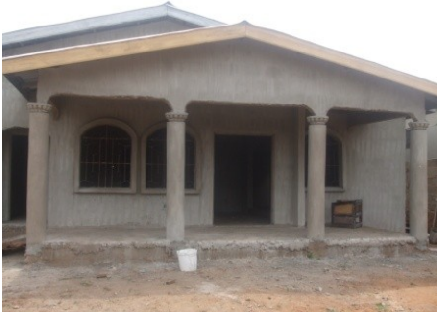
Plate 4.4: Plastering stage of the self-help housing process
