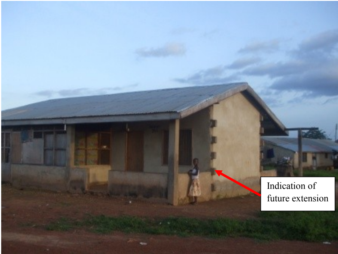
Plate 4.5: Core unit with indication of future extension
