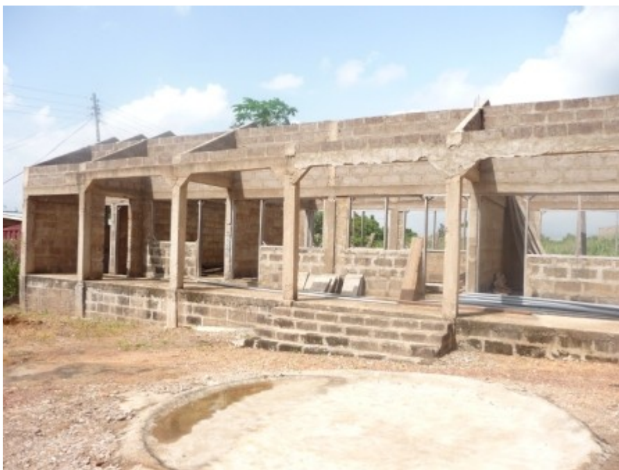
Plate 4.3: Completion of walls to gable level
