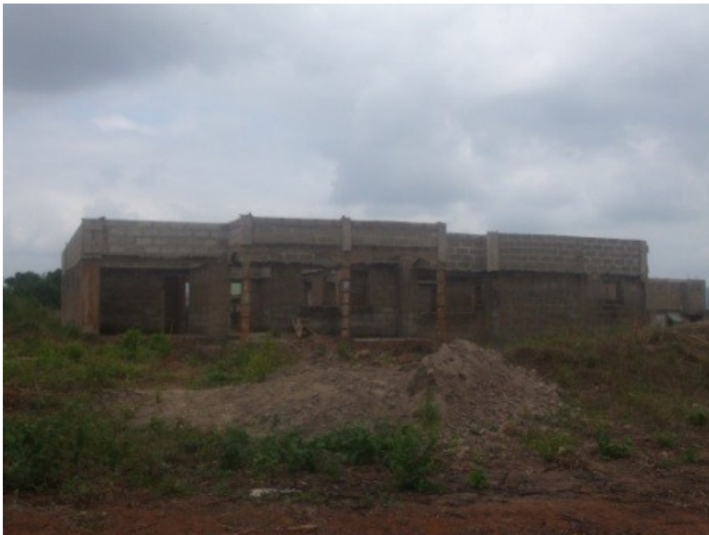
Plate 4.2: Construction of walls to lintel level
