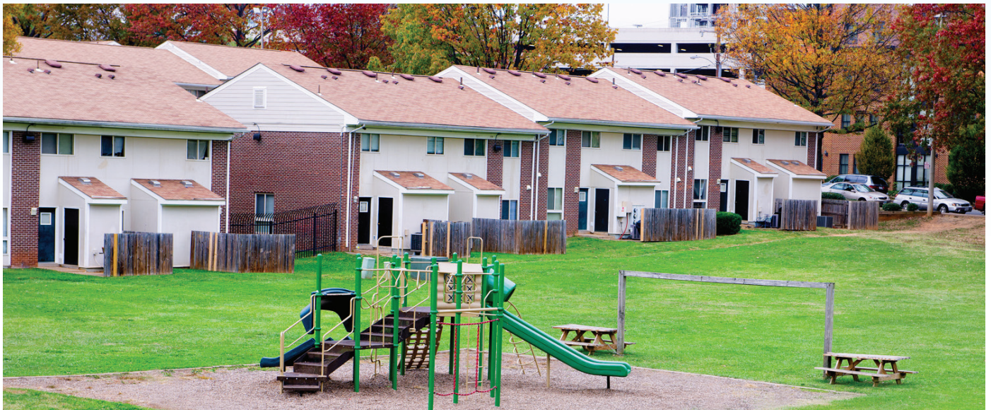
Friendship Court, Charlottesville, Virginia. NHT-Enterprise invested over $250,000 in high-efficiency HVAC systems, appliances, and lighting, reducing annual operating costs by $50,000.
