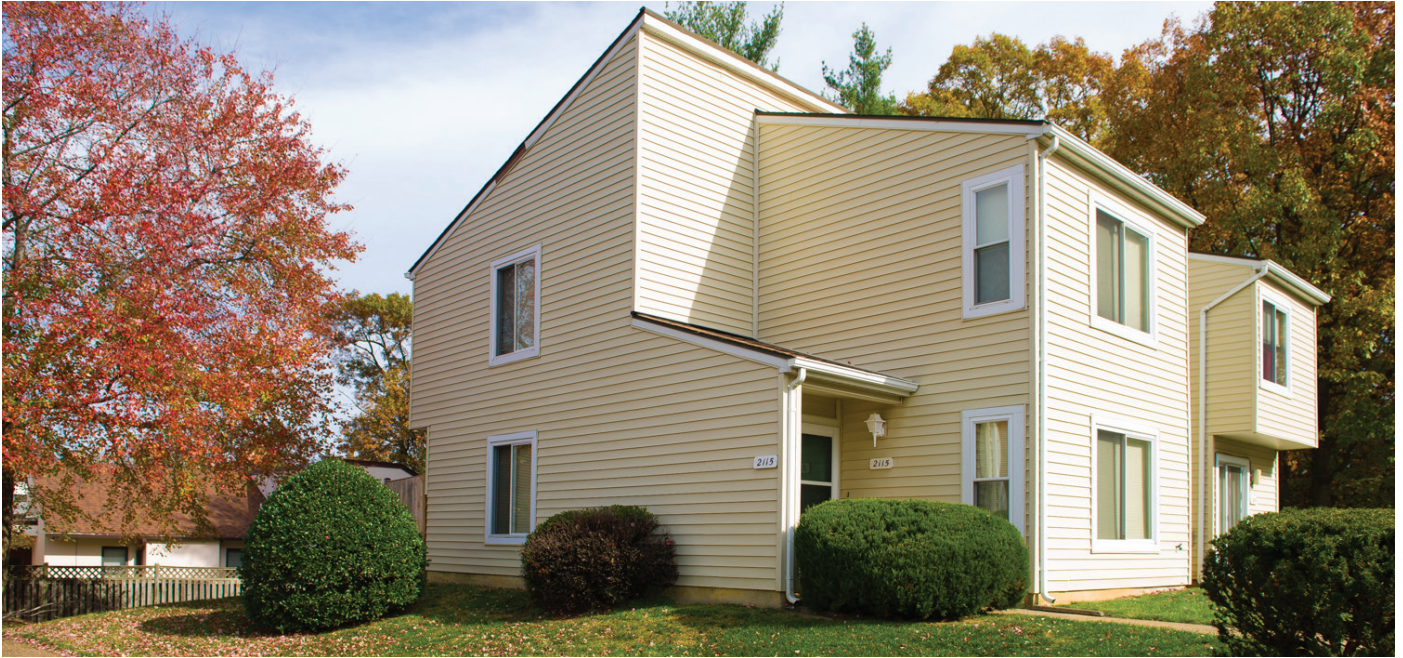
Briarcliff Apartments, Vienna, VA.
