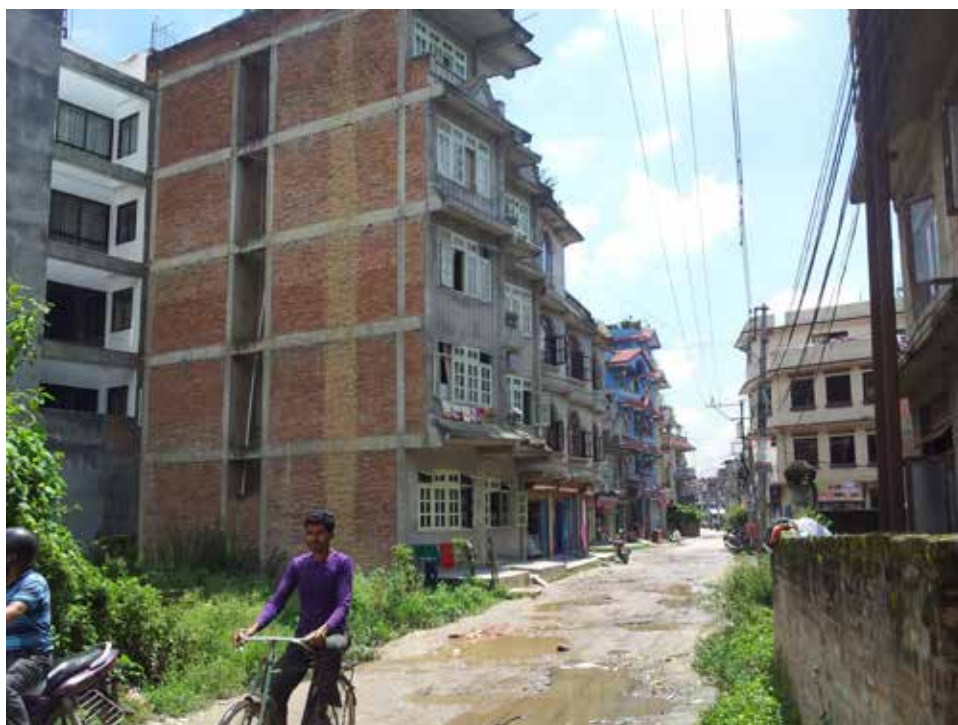
Figure 11. Examples of building bylaw violations in Khusibu
