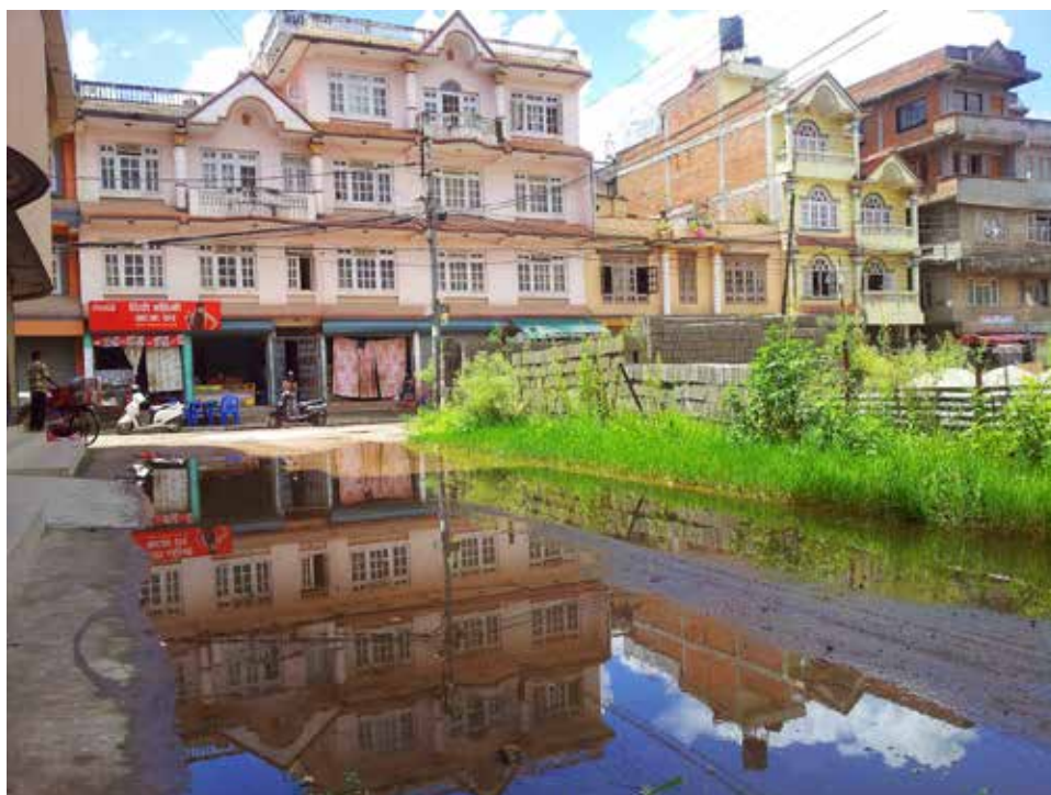
Figure 12. Drainage problems in Khusibu
