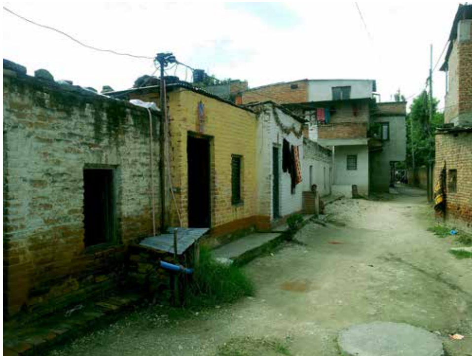
Figure 7. Concrete structures in Sankhamul
