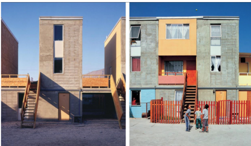
Housing designs by Elemental in Chile have enabled incomplete, low-cost housing (left) to be delivered to low-income residents and completed by them over time (right). 23
