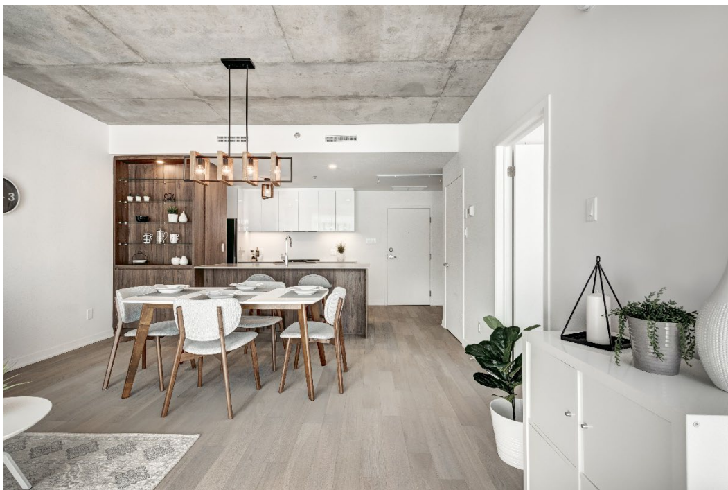
Figure 13: Indicative apartment interior with exposed concrete slab as the ceiling and surface-mounted light fittings.
