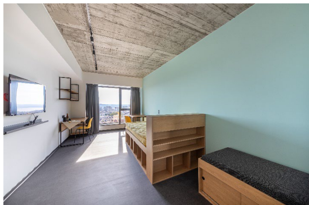
Figure 26: Example of exposed concrete slab (unpainted ceiling) finish in a student studio
