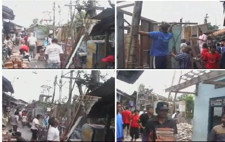
Figure 5.1 In Solo slum community dismantled their houses voluntarily because the city government provided them better living spaces (Habitat Day in Solo, 2007)
