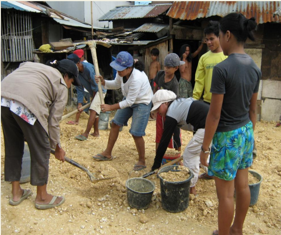
Communities in the Philippines building local infrastructure (Source: The Philippine Alliance, 2011)
