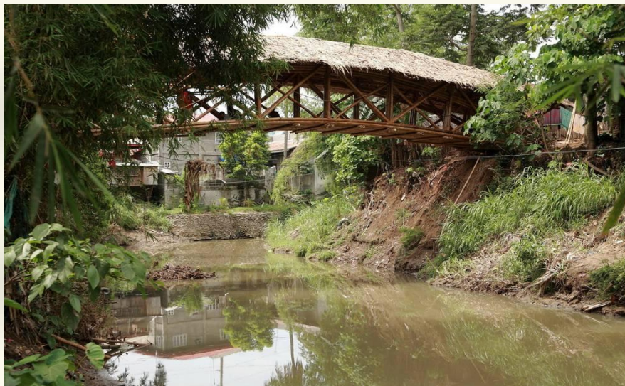
Before and after a community-led bridge building project in the Philippines (Source: Community Architect Network, 2011)
