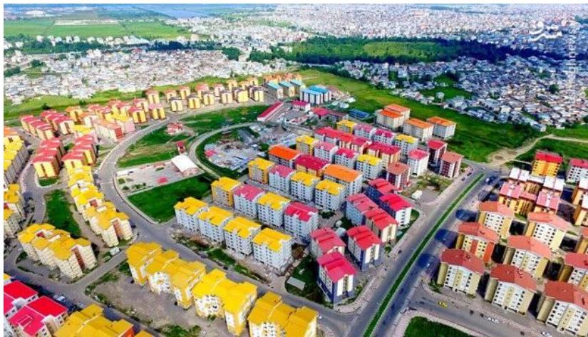
Figure D-2 Picture of Mehr housing units of Rasht
