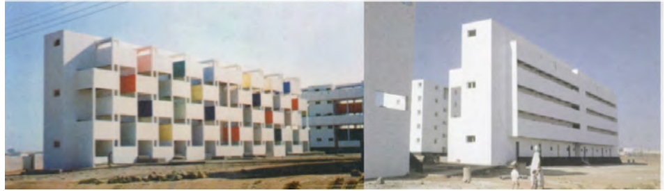
Figure 10. 'Nid d'Abeille': 'Checkerboard' south facade (left) and enclosed north facade (right)
