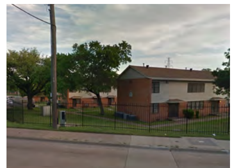
Aging public housing in close proximity to the station
