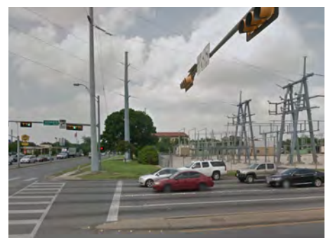
An electrical substation across Illinois Ave
