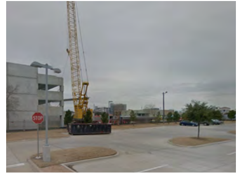
A currently-completed parking structure immediately adjacent to DART's parking lot
