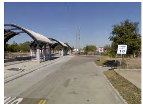
Trunk Ave., looking at the DART Rail station
