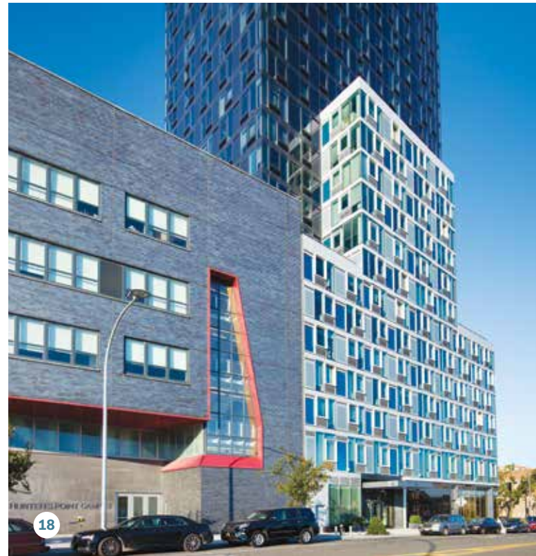
14. Windows and Doors: The SHoP-designed façade (visible here at the Crossing building) integrates HVAC units into window systems, incorporating the louver panels at the exterior, which streamlines the visual impact of the building system components.
