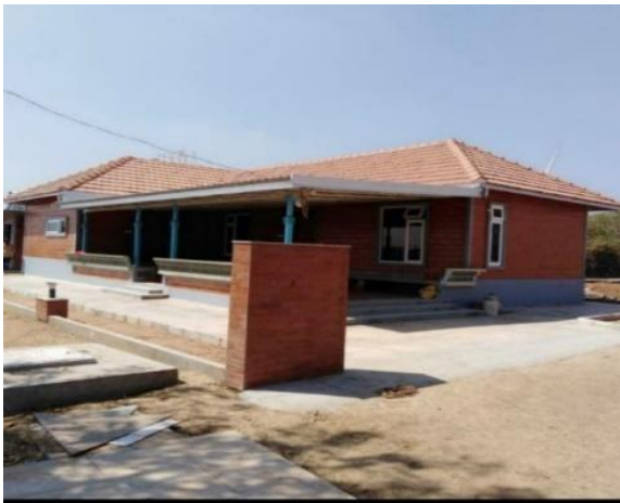
Figure 1. Ecofriendly Residential Building
