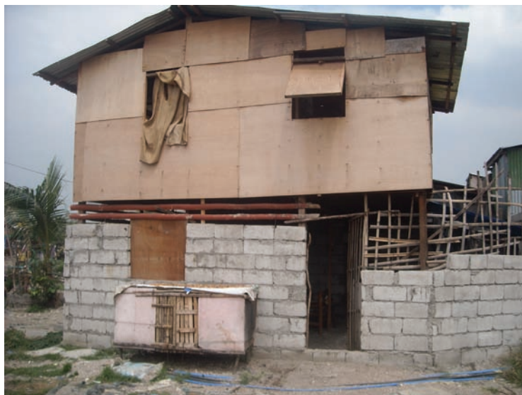
PHOTO 5 House constructed with ACCA support
