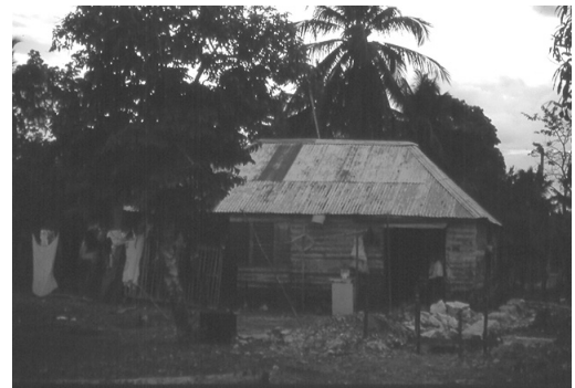
Figure 1: Typical Mayan house with previous thatch roof, substituted by a "modern" galvanized material.
