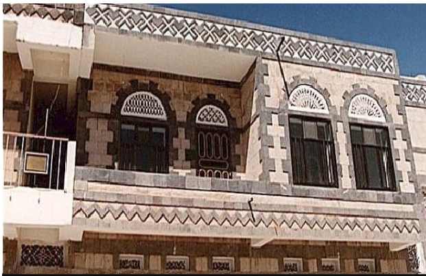
FIGURE I MODERN/TRADITIONAL CONSTRUCTION, REINFORCED CONCRETE FRAME WITH LOCAL STONES CLADDING (PICTURES WERE TAKEN BY AUTHORS IN 2011)
