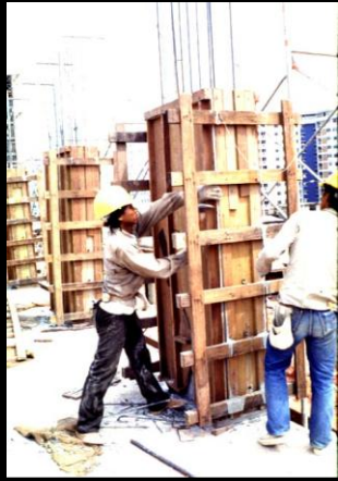
Extensive use of Timber formwork in early 1970s
