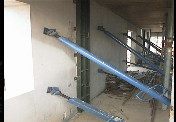
Minimal Metal formwork working in Tandem with Precast Technology in the 1990s
