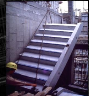
Precast Stair flights
