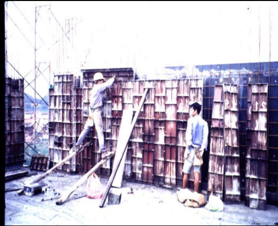
Extensive Use of Metal formwork in 1980s
