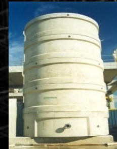
Segmented Water Tank
