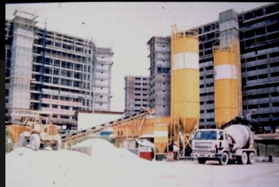
1980's - Semi-Automated Site Batching
