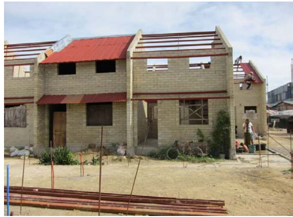
Figure 9. Community-designed and community-built houses in LTHAI by ACHR, 2011.
