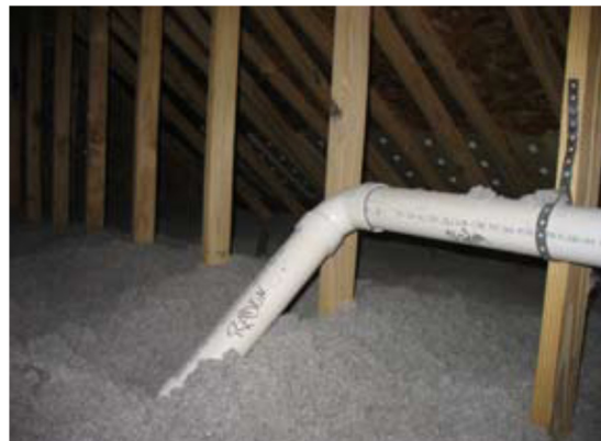
FIGURE 5. Improved ceiling insulation to R-38.
