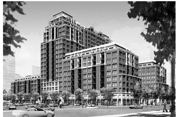
One Metropolitan Park Courtesy of: Arlington County Community Planning, Housing, and Development
