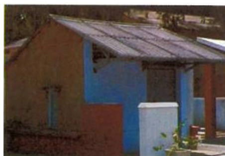
Fig. 1. Mud Plastered House
