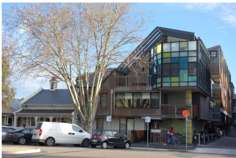
Figure 9: Photograph of PPHA’s Kyme Place affordable housing project
