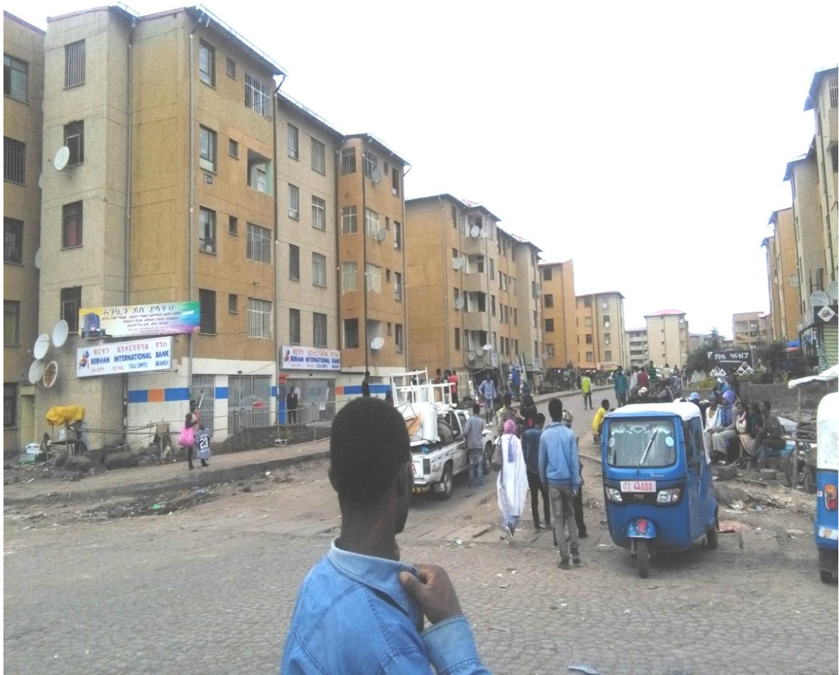
Figure 2.1 Tuludimtu condominium site (Source: compiled at field survey,2017)
