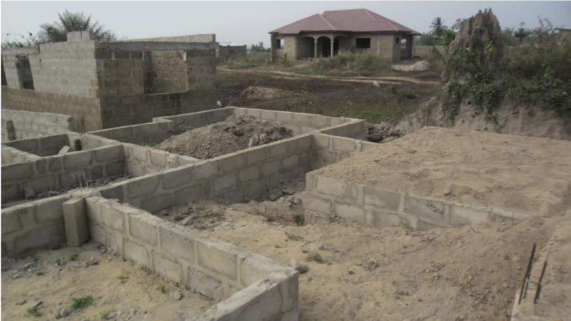
Figure 7: Foundation of a House. Source: Kas Estates, Ghana.com
