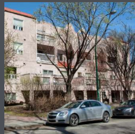
Before the renovation
