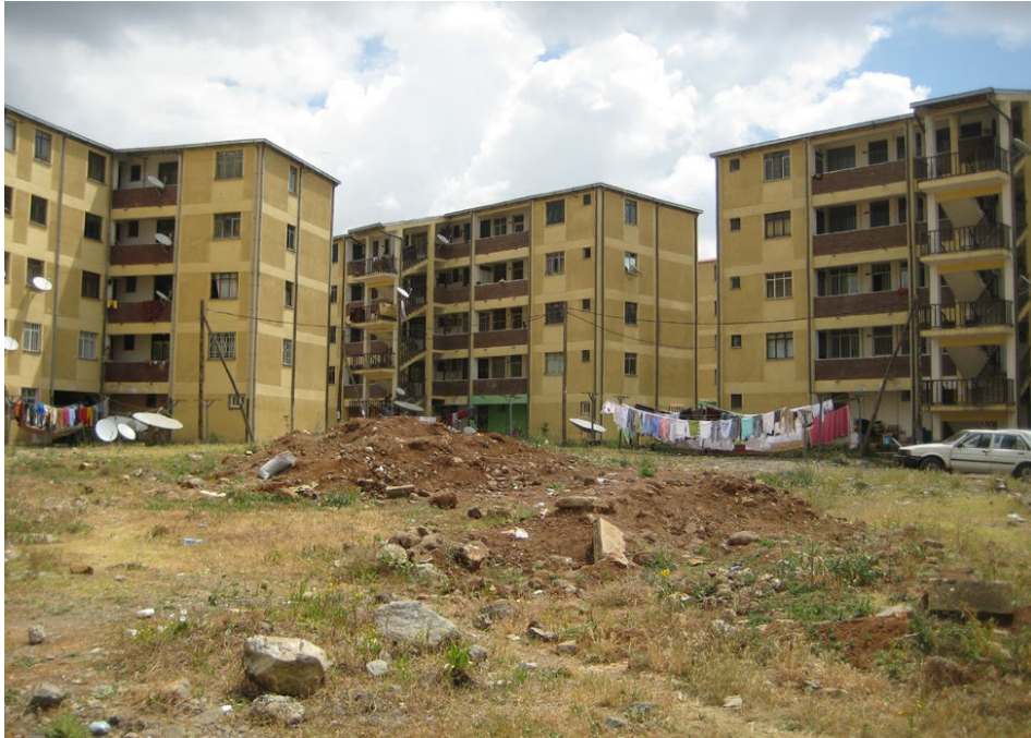
Stand-alone housing blocks with neglected outdoor spaces (source: author, 2011).
