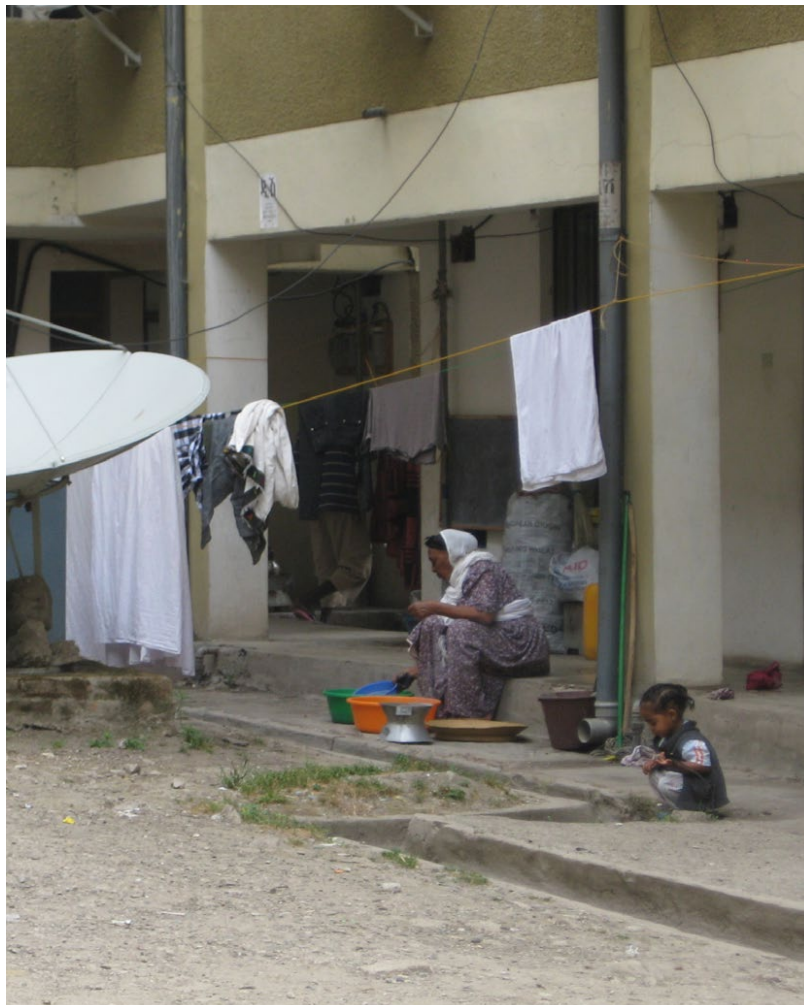
Immediate outdoor space appropriated by cooking, laundry, storage, and satellite dishes (source: author, 2011).
